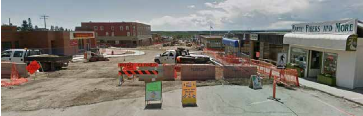
Figure 11 - Street revitalization construction (Google Street view, June 2014)
